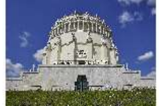
KeBf.I, Fassade, DI014259, BSV-
